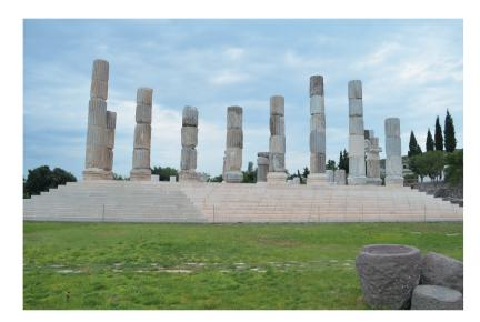
Figure 11. Re-erected original columns on new crepis on south-west side, Smintheion.
