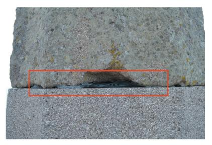
Figure 2. Lead plates between column drums, Assos.
