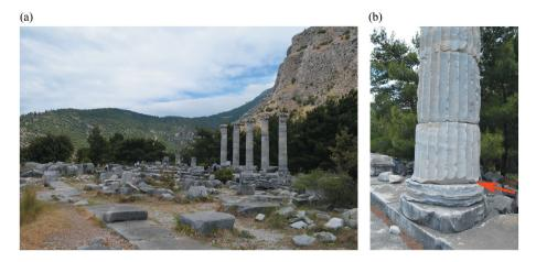
Figure 5. Re-erected columns of the Temple of Athena with reduced height in the sanctuary and missing torus, Priene.
