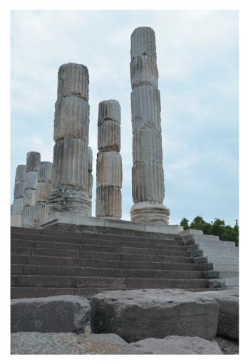
Figure 10. First erected three columns on re-built foundation and crepis on south-east side, Smintheion.
