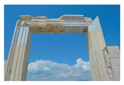
Figure 23. Completions of the door with different materials as marble and reinforced concrete at Laodikeia.
