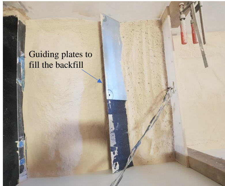
Figure 4.12. Preparing the backfill (Top view)
