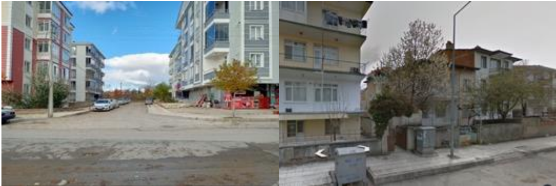
Figure 5. 3. Conditions of Building in Buharaevler (left) and Gülabibey (right) Neighborhoods.
