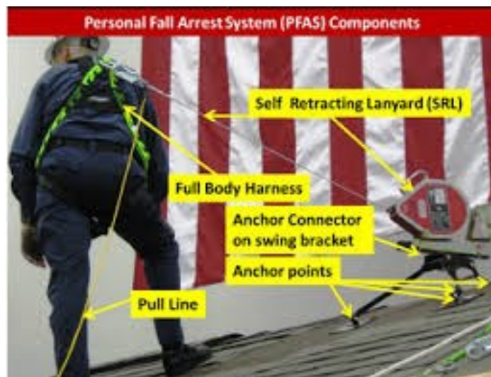
Figure 3.3. Basic Components of a Personal Fall Arrest System
