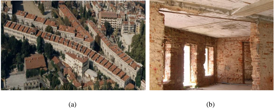
Figure 3.1. (a) General view of Akaretler Row Houses, (b) Load-bearing masonry walls and RC slabs of Akaretler Row Houses (Source: Ispir, 2010).
