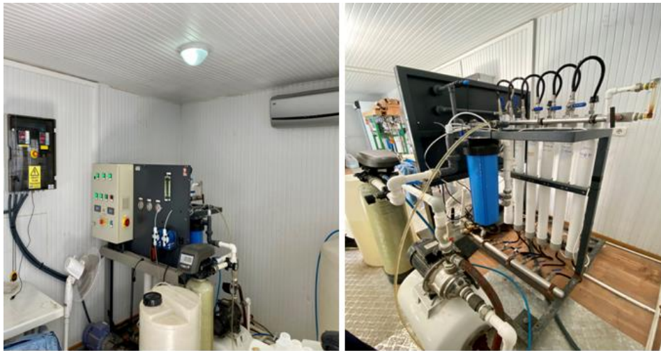
Figure 6.1. Front and back view of RO membrane system.
