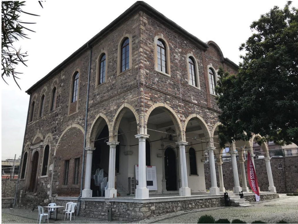
Figure 4.14. Exterior of the church (11.10.2019)
