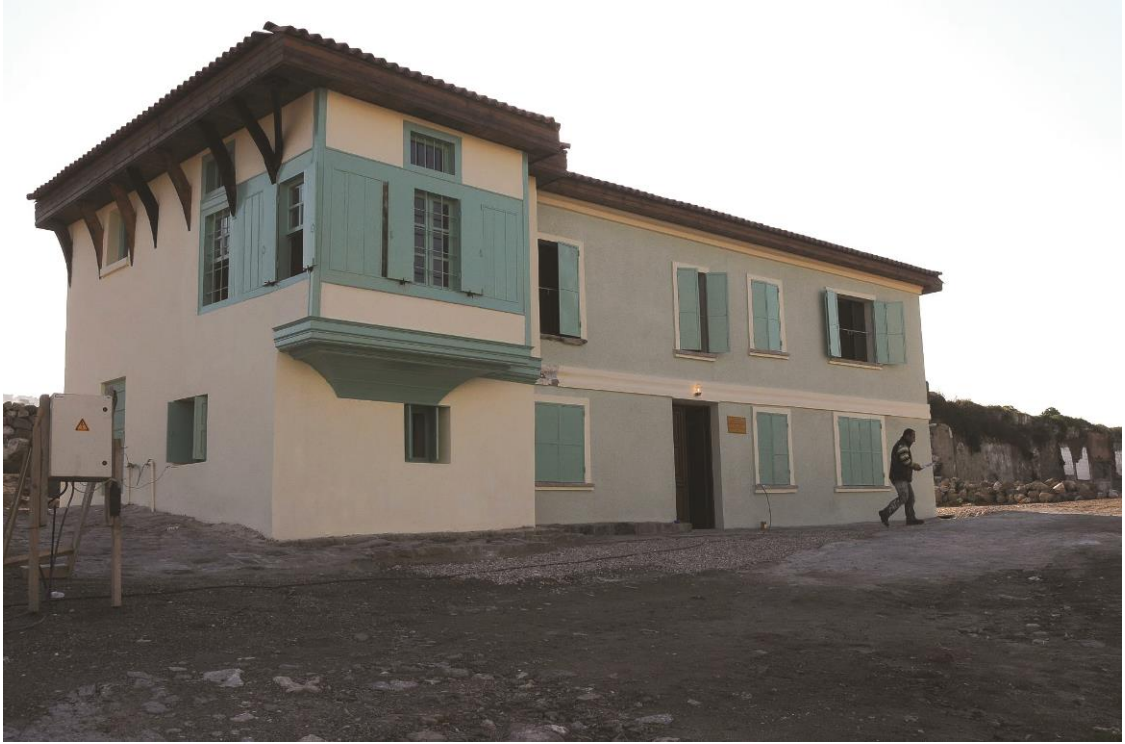
Figure B.B. 31. The excavation house (Source: Metropolitan Municipality of İzmir)
