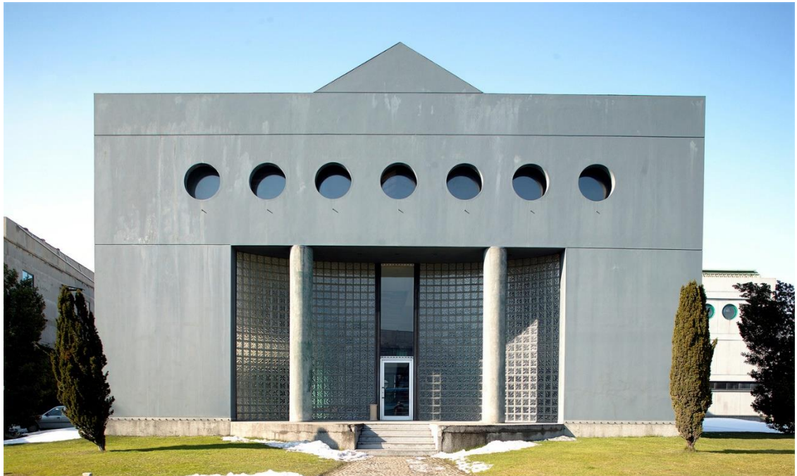
Figure 5.1. The front façade of Gön Leather Factory-1 (Source: “Nevzat Sayın - NSMH”, 2022)
