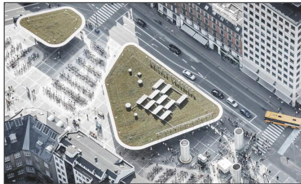
Figure 3.13. Green roof of the station (Source: https://cobe.dk/place/norreport-station )
