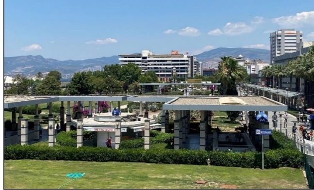
Figure 4.11. Konak metro station area
