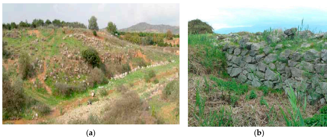
Figure 4. Mycenaean anti-flood dams: (a) General view of Tiryns dam (photo A. N. Angelakis) and (b) Cyclopean anti-flooding wall in Kopais (photo [35]).
