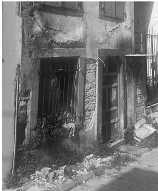
Figure 12. Postane Street House Nr: 10, S-Type, natural stone walls.
