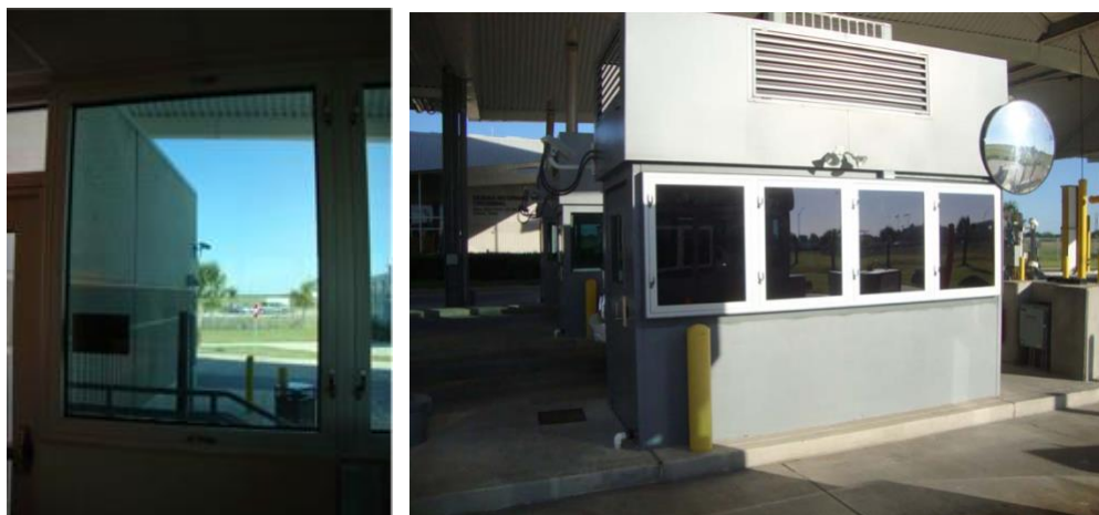
Figure 2.3. Tinted glazing used for the experiment in Donna Land Port (Source: Luis et al. 2015)
