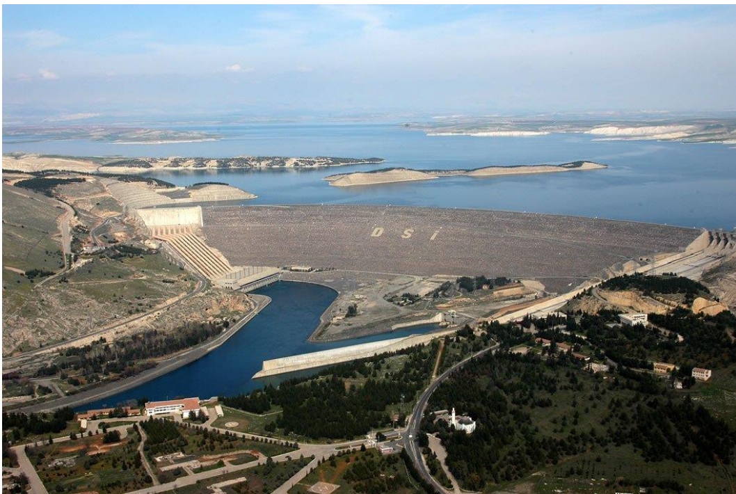
Figure 1.2 Atatürk Dam (Source: ataturkbaraji.com )
