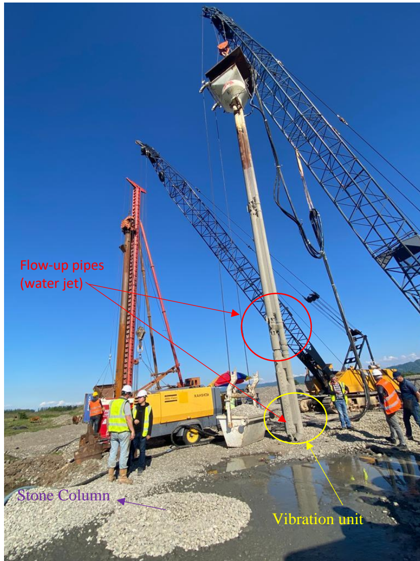
Figure 2.7 Wet–bottom–feed method rig and constructed stone column (Georgia, 2023)
