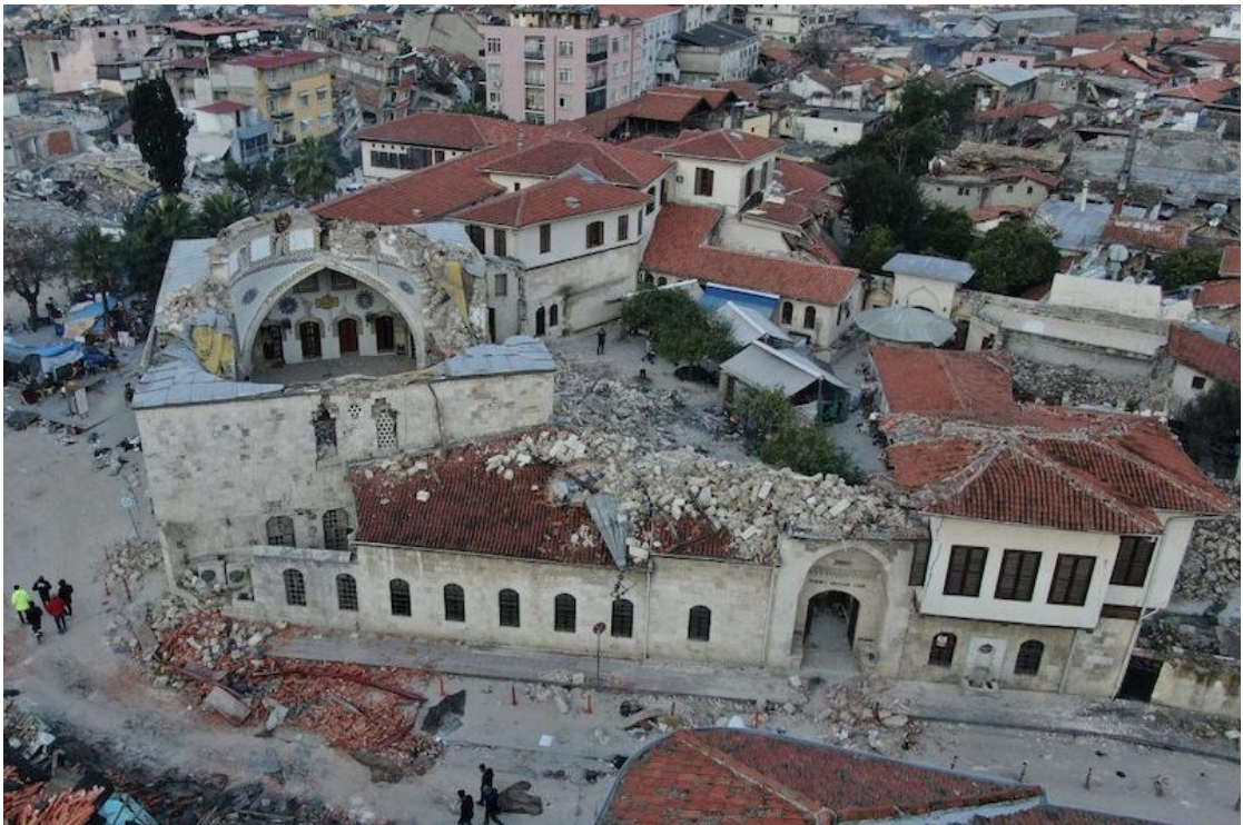
Figure 3. 34. Habib-i Neccar Mosque after February 6, 2023, Pazarcık and Elbistan earthquakes (Source: Arkeofili 2023)
