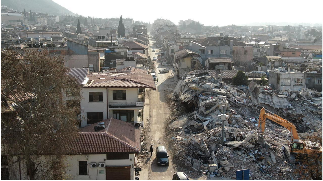
Figure 3. 35. Kurtuluş Street after February 6, 2023, Pazarcık and Elbistan earthquakes (Source: TRT Haber 2023b)
