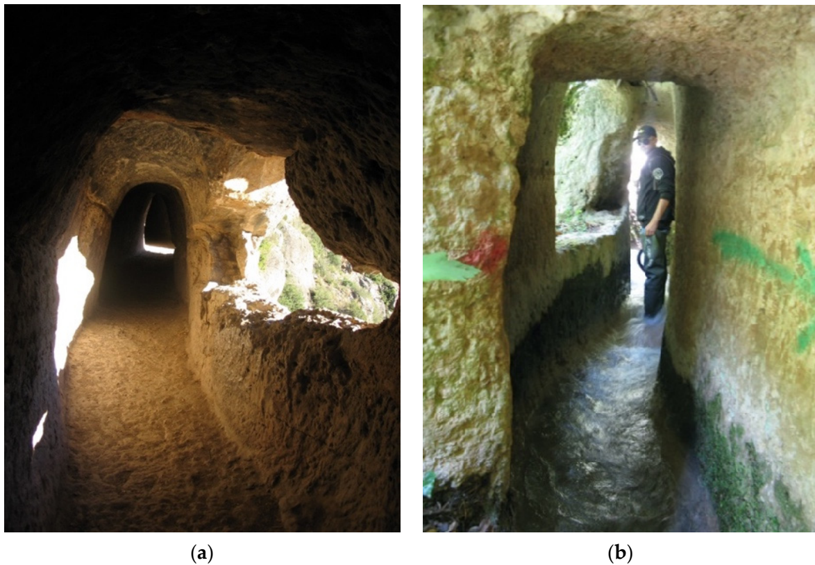
Figure 18. Valley-side tunnels with “windows” from which the tunnel was excavated: (a) Chaves aqueduct, Spain, and (b) Galermi aqueduct, Sicily (Photo Cees Passchier).
