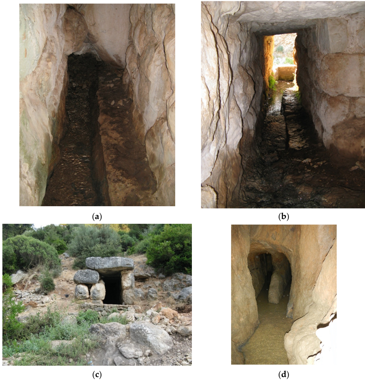
Figure 12. Spring tunnel of the Xanthos aqueduct, Turkey. The tunnel was partially dug into the rock and extended with ashlar and cover stones. The channel is deepened, leaving a footpath along the side for access: (a) inside, looking to the exterior; (b) inside, looking towards the spring; (c) exterior. The structure is still in use to provide water for irrigation. (d) Branching tunnel of Novalja, Croatia. The tunnel was bifurcated to access two springs (Photos Cees Passchier).
