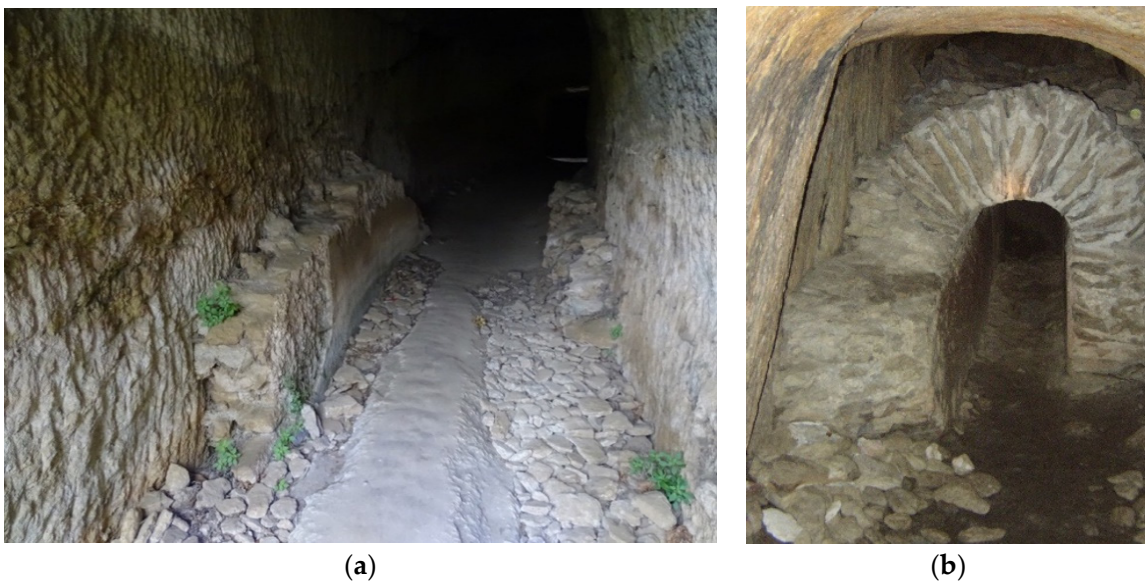
Figure 16. Conduits built into an aqueduct tunnel: (a) Sernhac tunnel, France; a masonry channel was built into the tunnel for passage of the Nîmes aqueduct (Photo (a)—Cees Passchier). (b) Cave de Curée, with a vaulted aqueduct channel in the tunnel, part of the Gier aqueduct of Lyon, France—( http://www.romanaqueducts.info/ , accessed on 15 August 2023).
