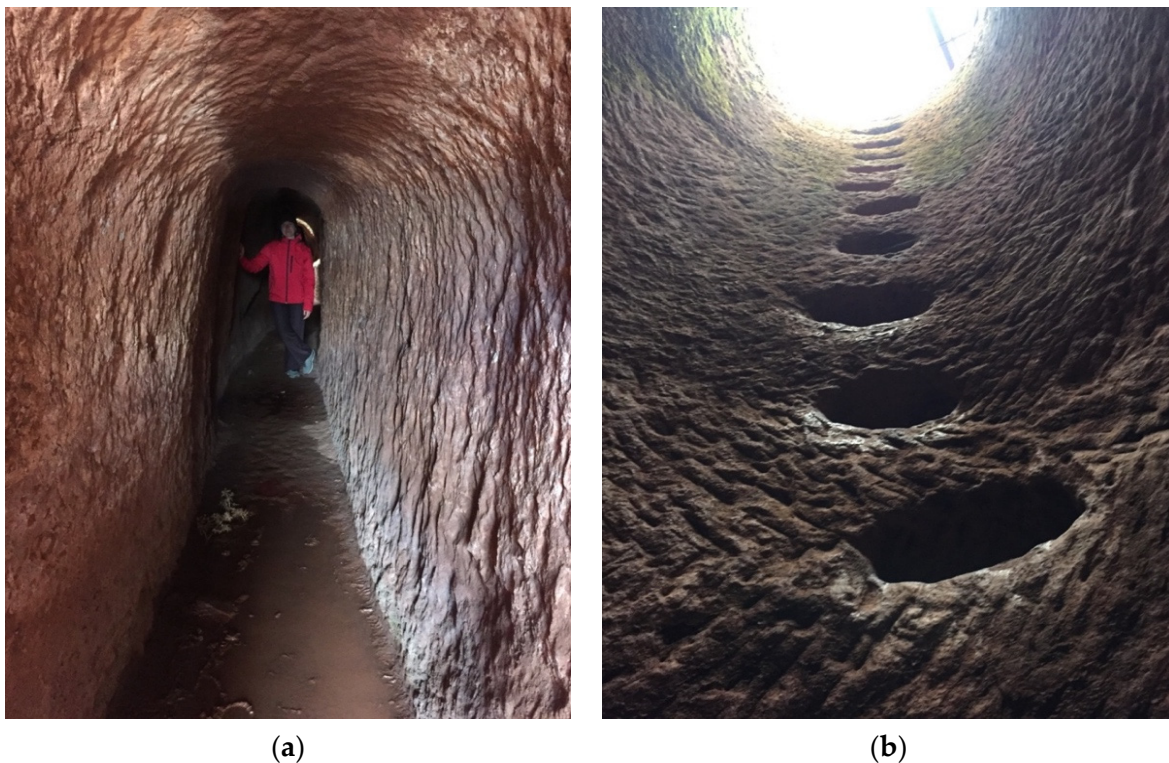
Figure 13. Qanat-mode tunnels and shafts: (a) tunnel and (b) vertical access and building shaft with niches for working crews, Tiermes, Spain (Photos Cees Passchier).
