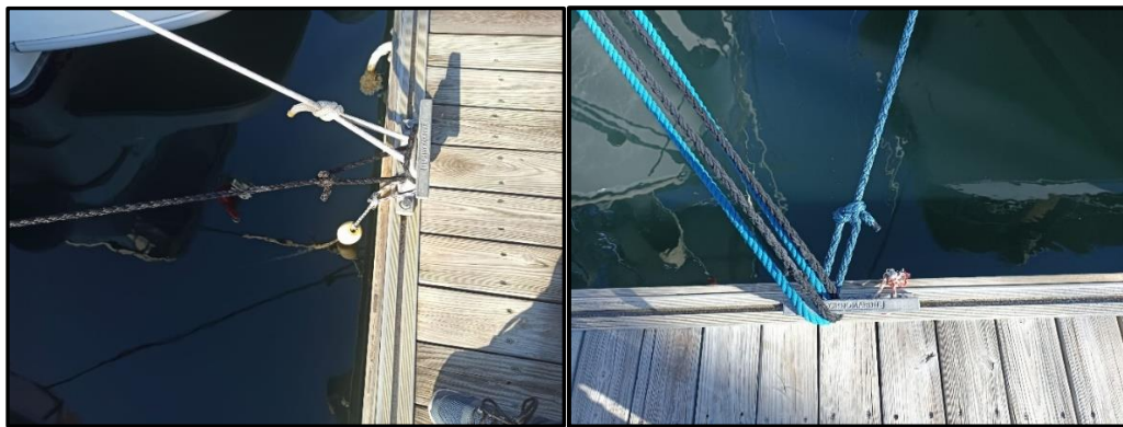
Figure 3.36. The cleats on the aluminum dock.
