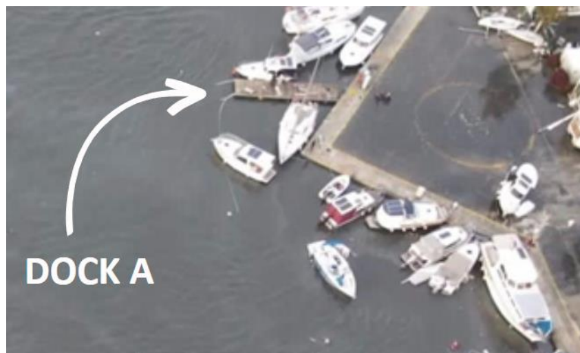
Figure 5.6. Remaining the pontoon of dock A after the tsunami.
