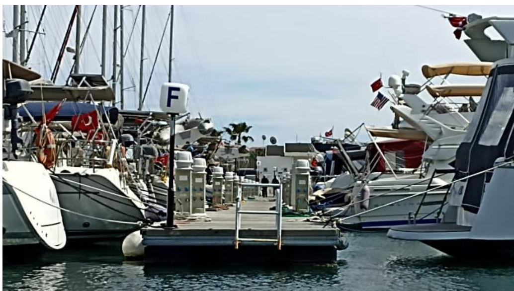
Figure 3.15. Dock F from the sea side.
