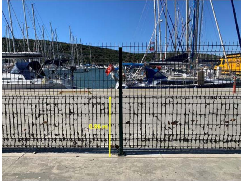
Figure 2.2. Tsunami marks on the garden fence in Teos Marina (Source: Doğan et al., 2020).
