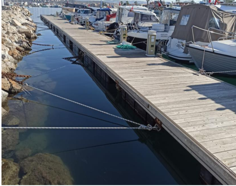
Figure 3.16. Repaired Dock with aluminum pontoons.
