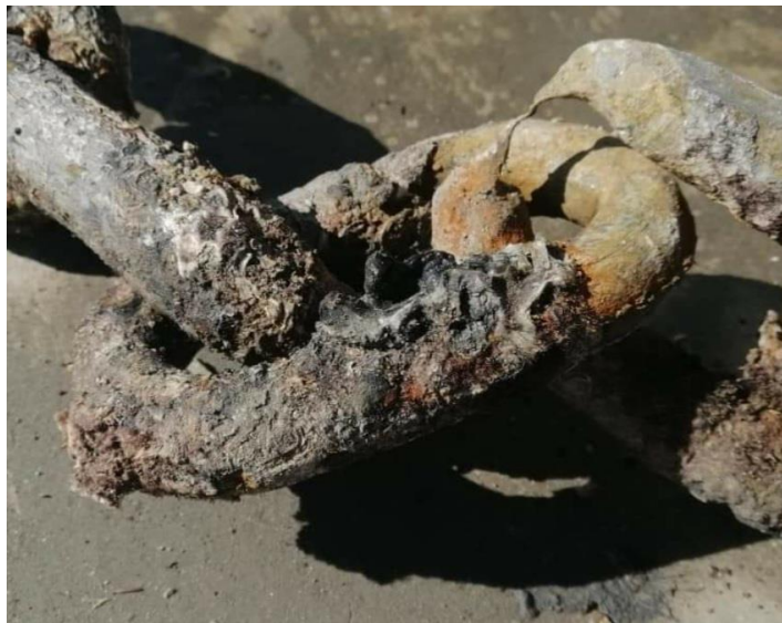
Figure 2.3. Broken chain in Teos Marina due to the tsunami.
