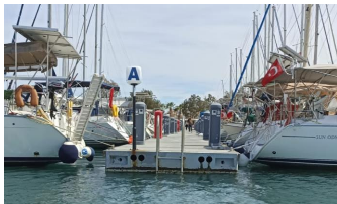
Figure 3.11. Renewed pontoon A after the tsunami.
