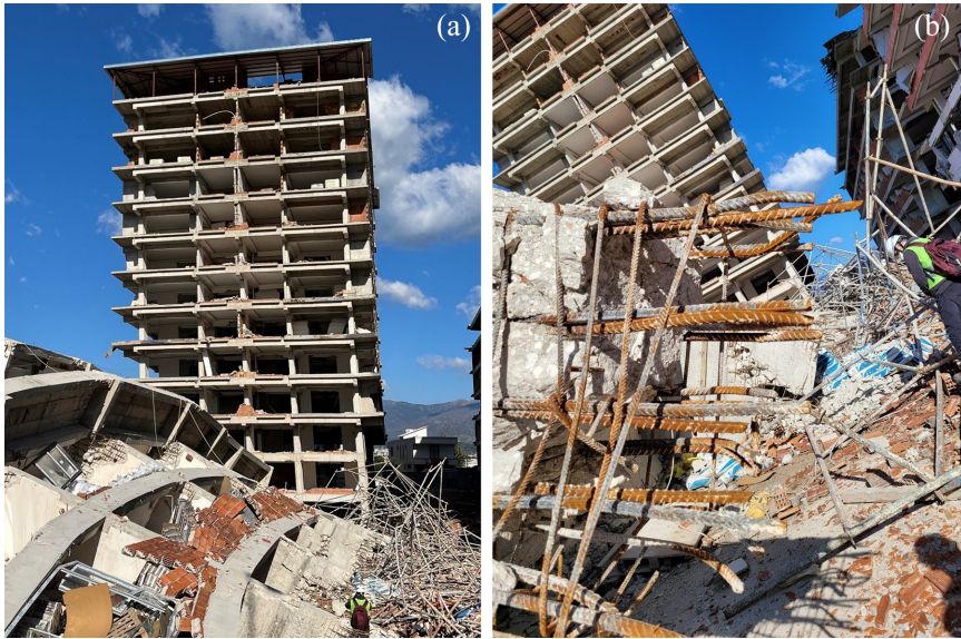
Figure 15. Building complex in Antakya: (a) building complex still standing with an approximate residual drift of 6% in the first story, and (b) identical structure that had collapsed (seen in the foreground of Figure 15a)
