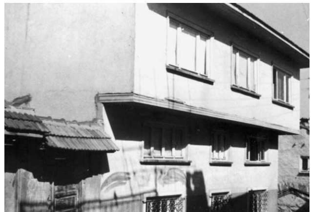
Fig. 6. A house in group "D".
