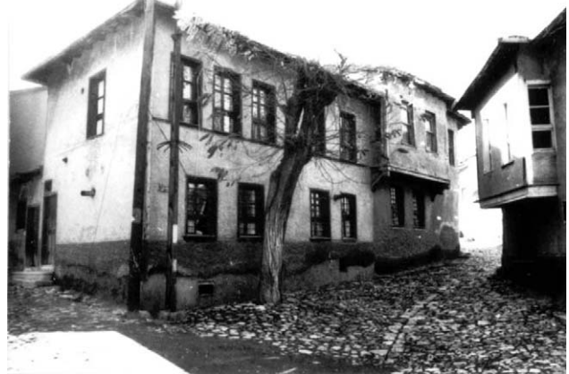
Fig. 1. Traditional houses give important vistas.
