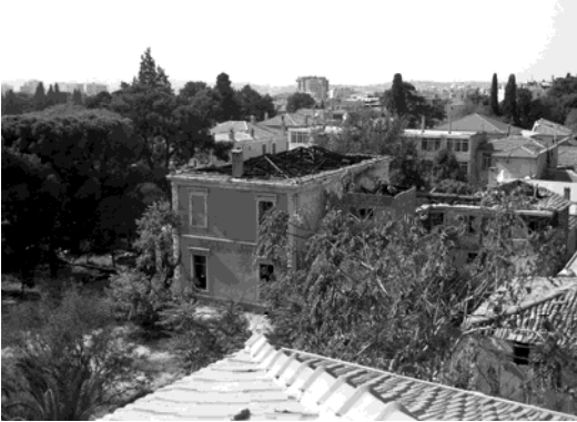
Figure 1 General view, Levantine House
