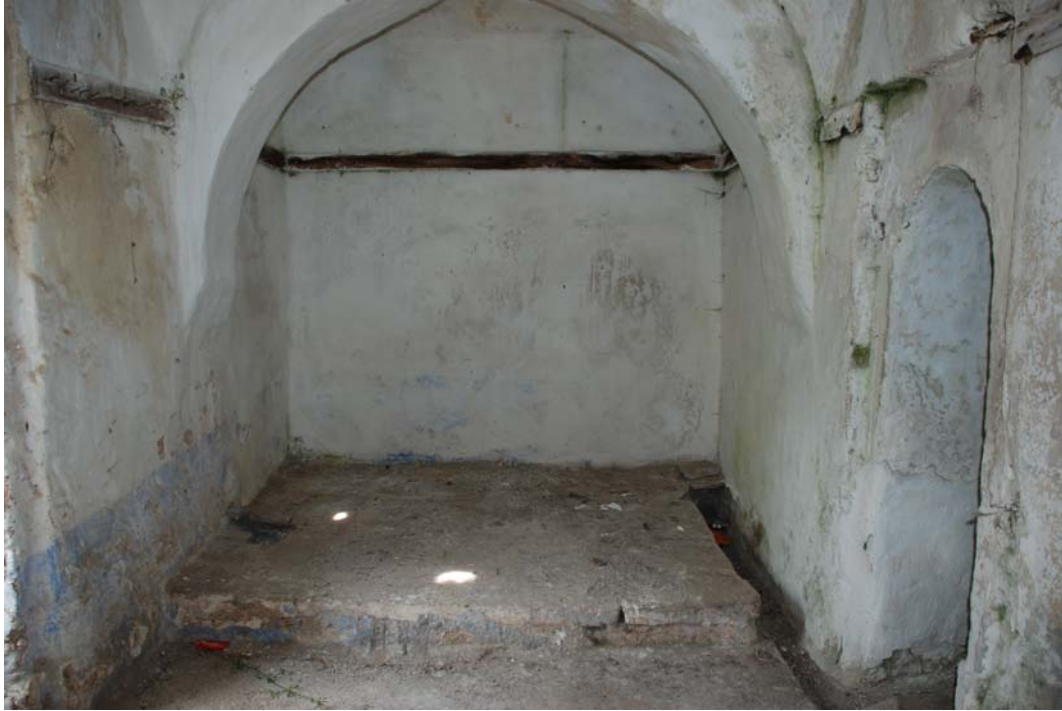
Figure 3.8. Northwest iwan in the main sıcaklık space.
