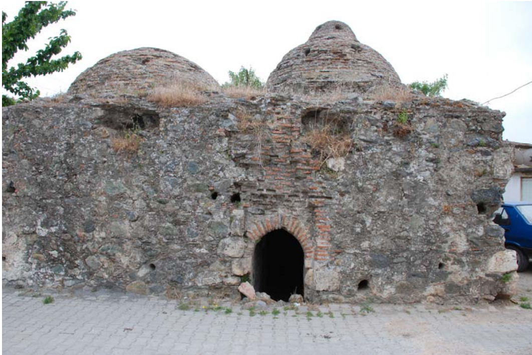
Figure 3.32. Depressed pointed arched door with yaşmak .
