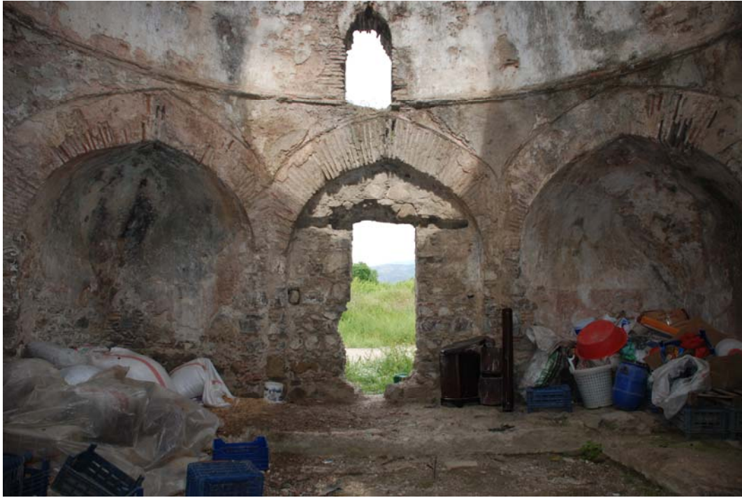
Figure 3.36. East wall of soynmalık space.
