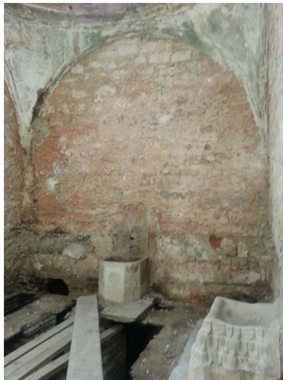
Figure 3.25. Wash basins in the southeast halvet .
