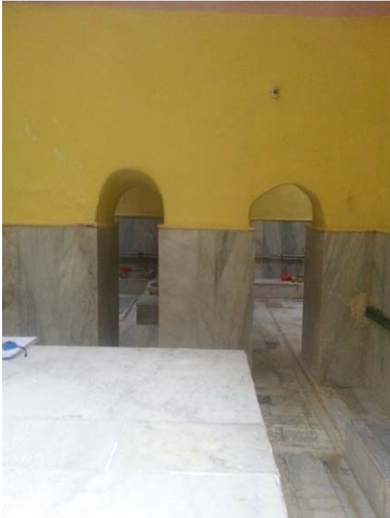
Figure 3.18. Door openings in the sicaklık .
