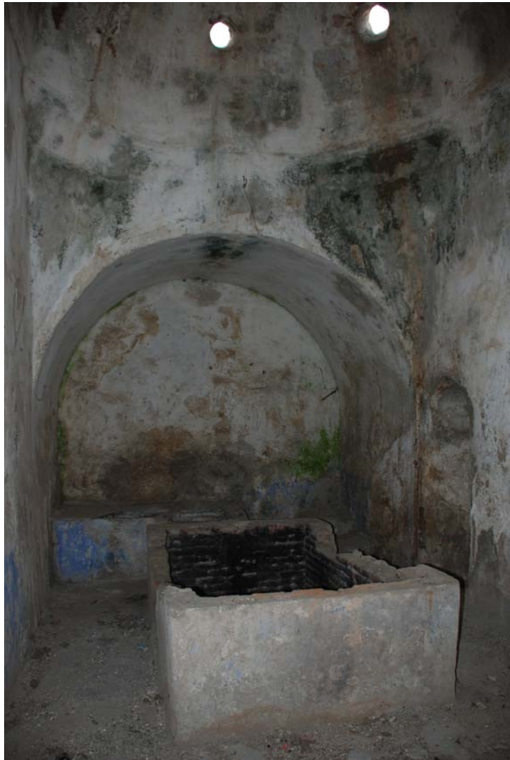
Figure 3.47. Western iwan and belly stone in the main sıcaklık .
