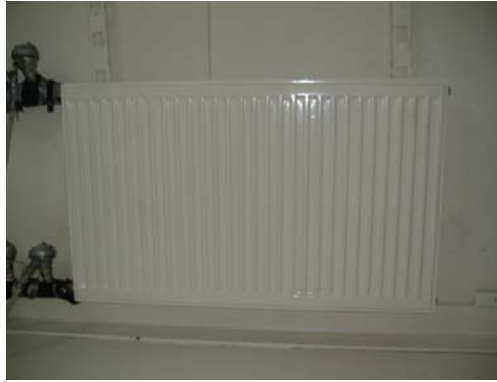
Figure 5.2. Placement of a radiator during a test procedure.
