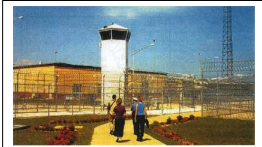
Figure 4.25 Wabash Prison Outside View
