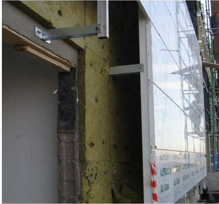
Figure 3.11. External Wall of ADM Building.
