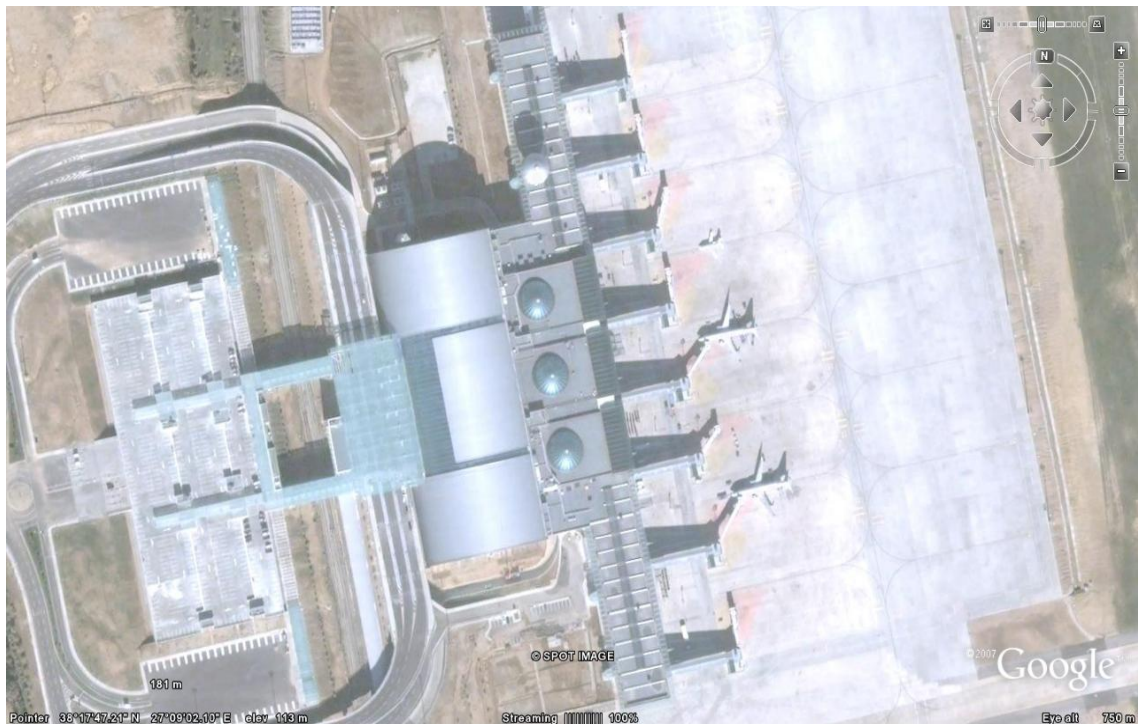
Figure 2.1. ADM Building Birds Eye View from Google-Earth.
