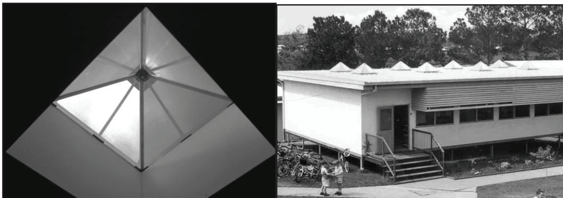
Figure 5.2. Views of skylight with lasercut panels
