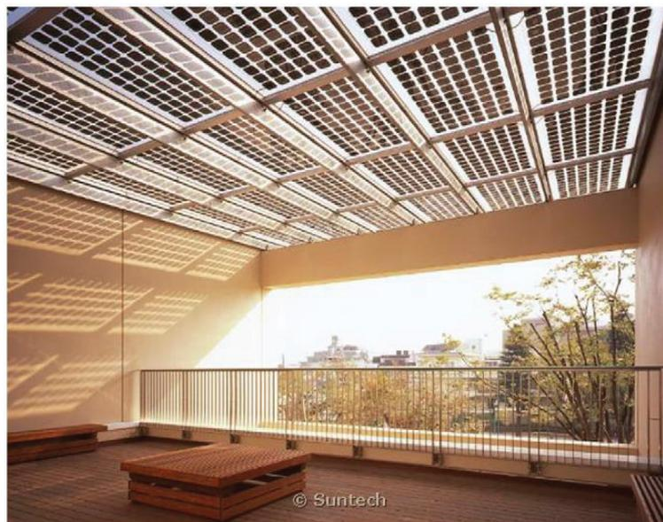
Figure 5.7. BIPV modules in the ceiling system
