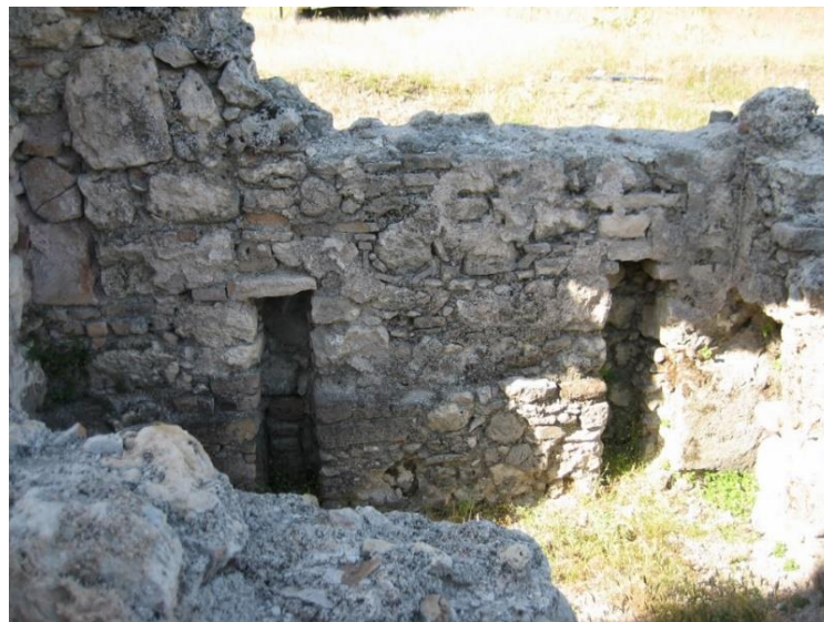
Figure 3.12. Space 3, southern wall
