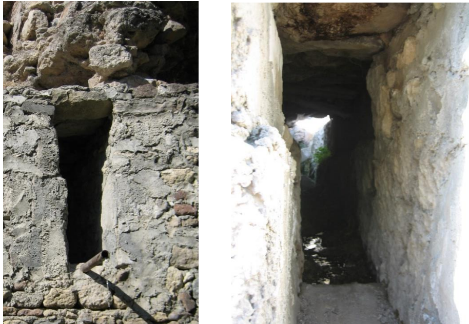
Figure 3.23. Water channel remain, exterior view from northeastern façade (left), interior view from space 6 (right)
