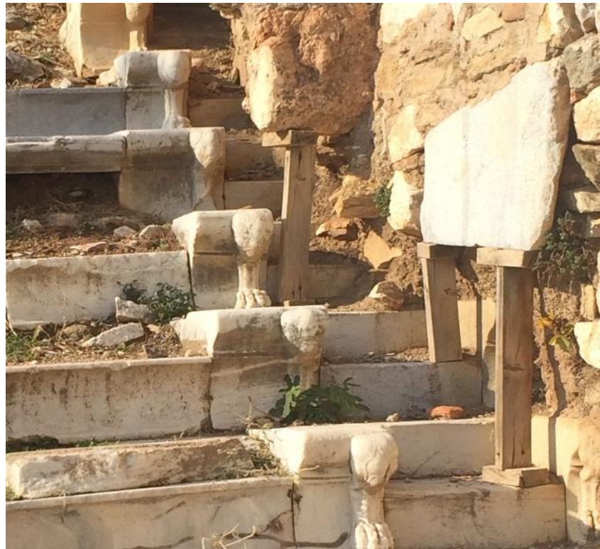
Figure 2.28. Supporting of the walls in the Bouleuterion, Metropolis
