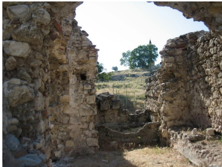
Figure 3.13. View from entrance to space 4
