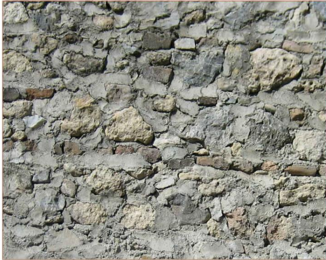
b. Load bearing wall: Rough cut stone with cement mortar
