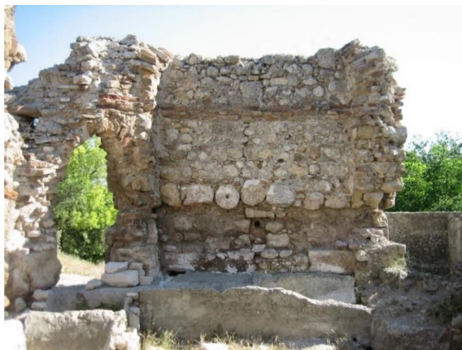
Figure 3.15. Space 6, as viewed from south
