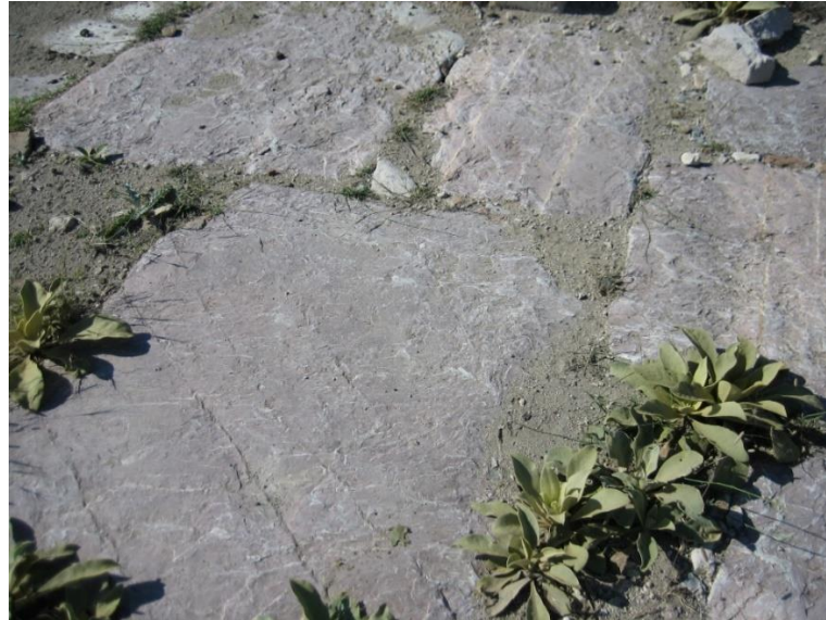
Figure 3.22. Stone floor covering
