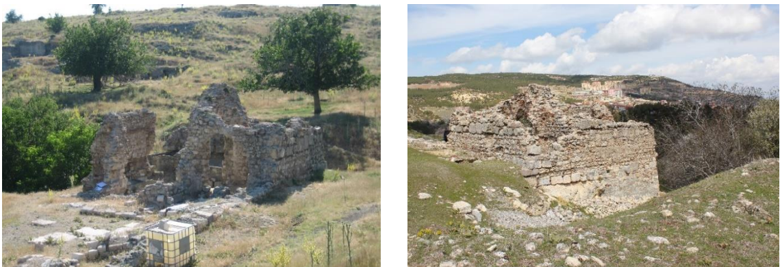
Figure 3.7. West façade (left), south façade (right)
