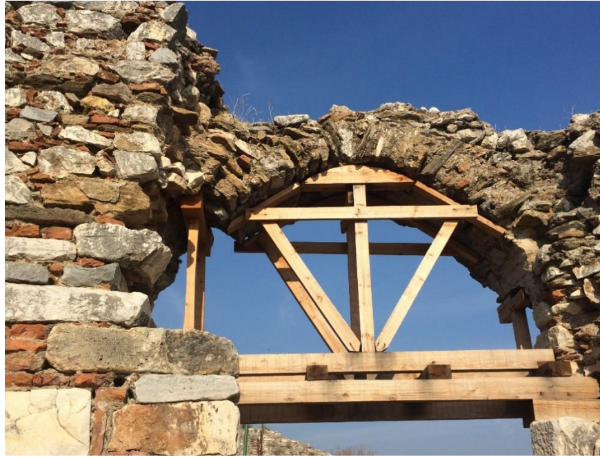
Figure 2.27. Consolidation of an arch in the Bouleuterion, Metropolis
