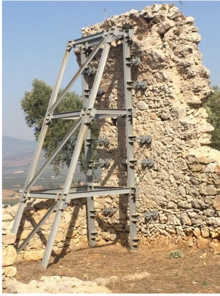
Figure 2.29. Structural interventions in Beçin Castle
