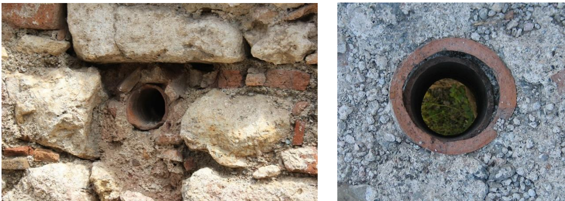
Figure 3.21. Horizontal pipe in space 4 (left), vertical pipe in space 6 (right)
