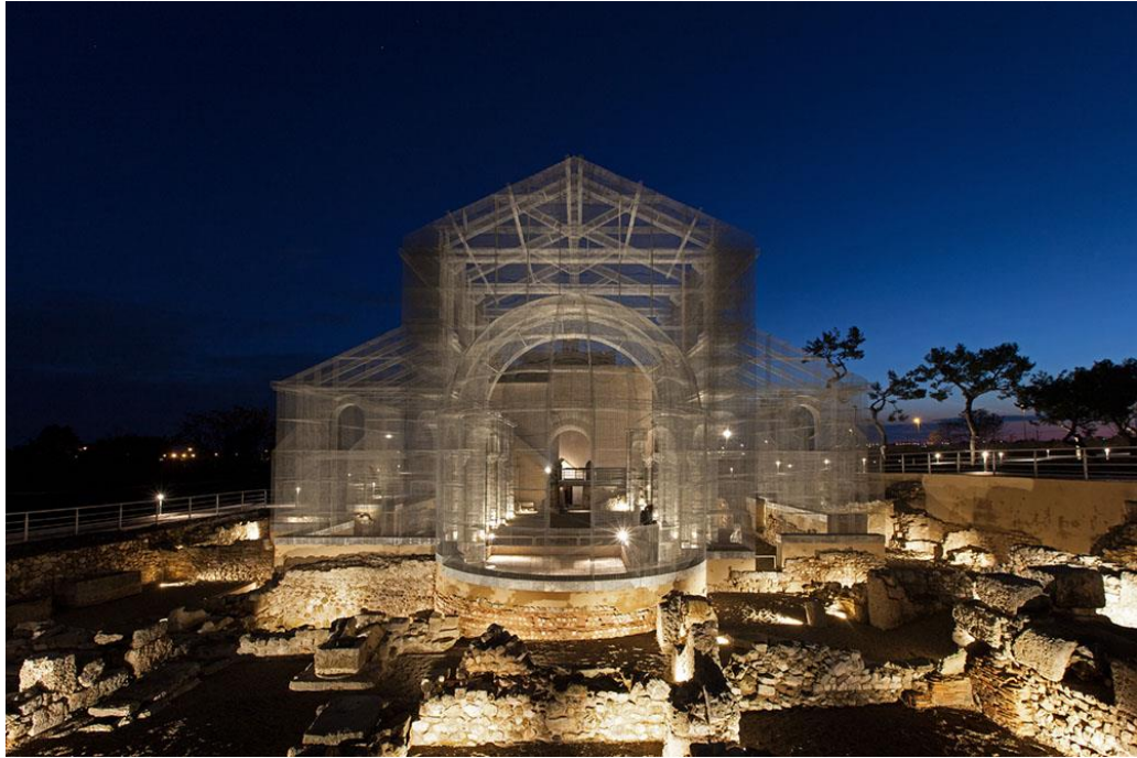
Figure 2.12. Basilica, after 2016 restoration (Source: Sierzputowski, 2017)
