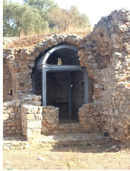
Figure 2.29. Structural interventions in Beçin Castle
