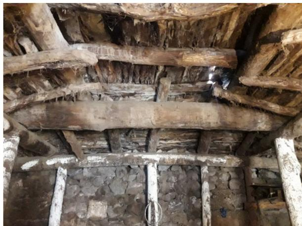
Figure 3.83. The west wall and corbelled ceiling of the southern part.
