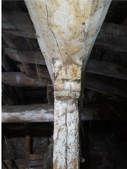
Figure 3.92. The merge of wooden capital and ceiling joist.
