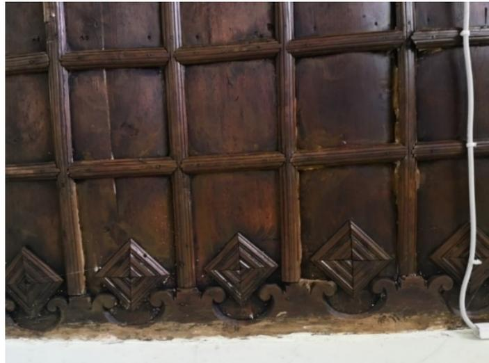
Figure 3.38. Detail of the mergence of daily room ceiling with the wall.
