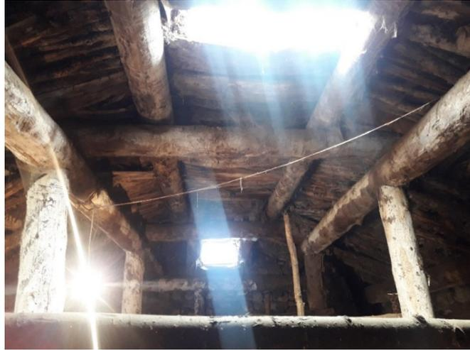
Figure 3.84. Corbelled ceiling and skylight of the northern part.
