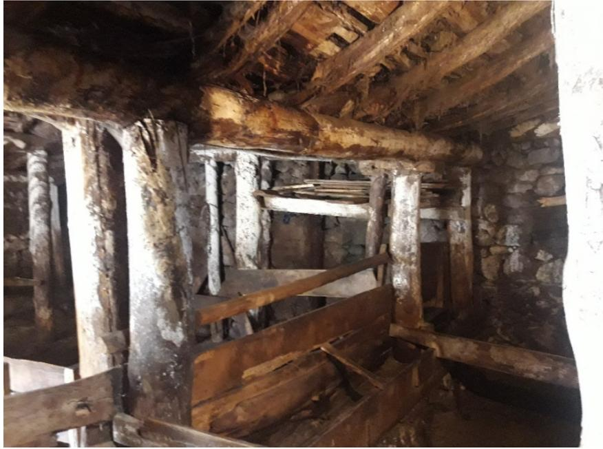
Figure 3.79. Serial of wooden posts separating the northern and southern parts.
