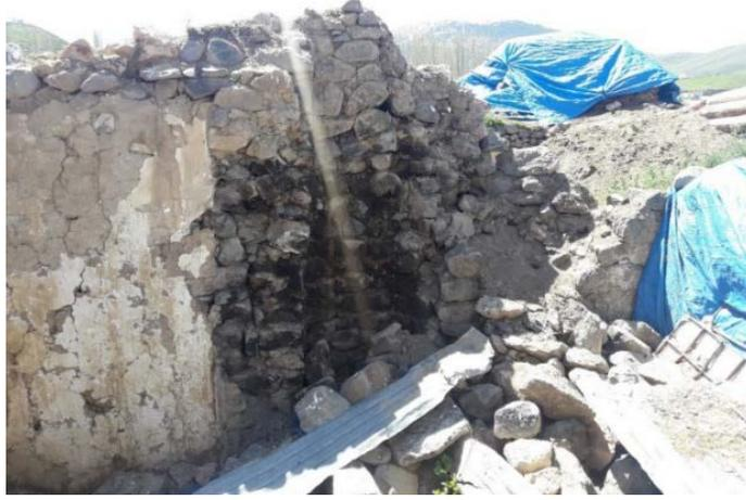
Figure 3.100. The ruins of the fireplace on the south wall of the machine house.
