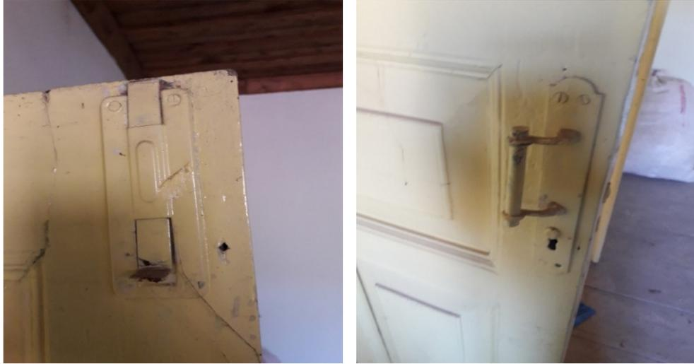
Figure 3.25. Metal bolt and door handle
