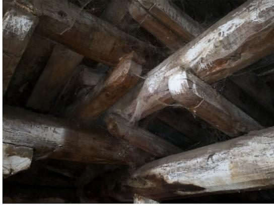
Figure 3.95. The corner merge of hammerhead joists.
