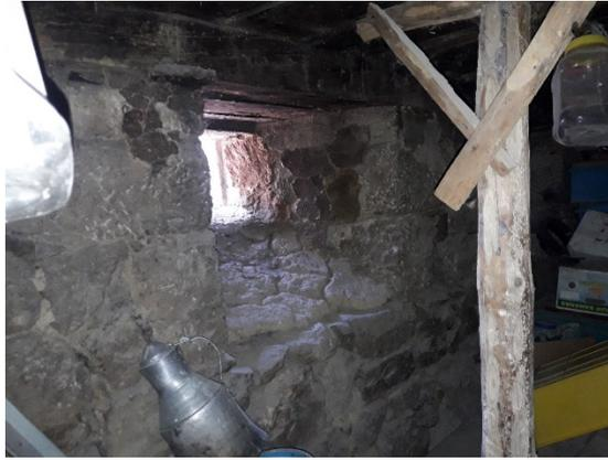
Figure 4.13. Wooden posts supporting the warehouse roof.
