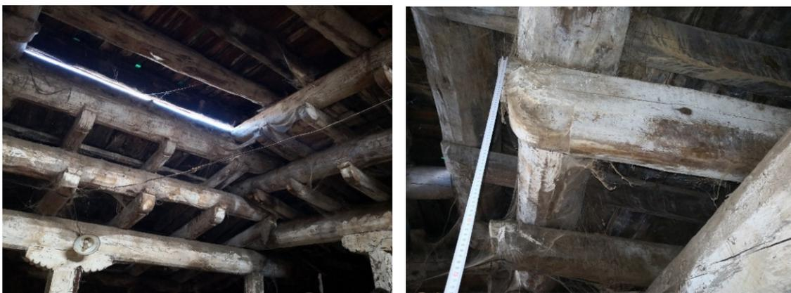
Figure 3.93. Corbelled ceiling and skylight and wooden joist sharpened in the form of hammerhead its ends (Photograph: Author, 2019).
