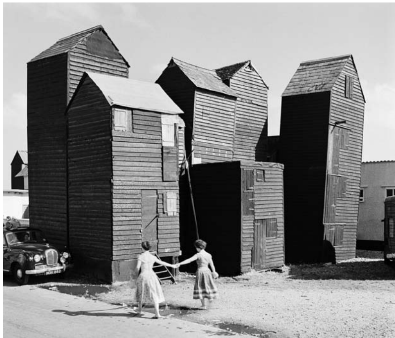
8.6 Two views of a group of fishermen's net shelters in Hastings, Sussex. Photograph by Eric de Maré, 1956, reproduced in The Architectural Review's article on 'the Functional Tradition', September 1957; The Architectural Review cover of March 1962 by Gordon Cullen.
